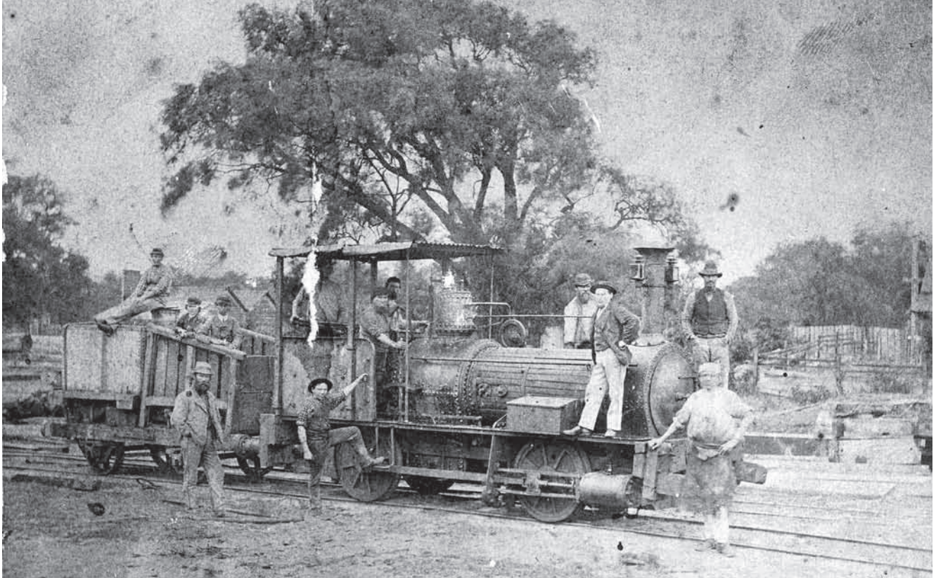
BALLAARAT in operation with an early home-built tender. This was later replaced by a more sophisticated metal-bodied example, though the under frame was timber. A hand coloured version of this image is on display at the Railway Museum in Bassendean, and cites the date as 1875. Photo: WAGR
