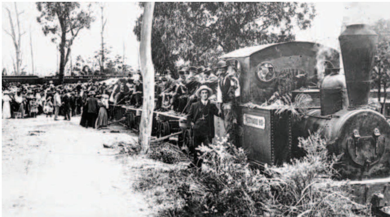
Bagnall 2-4-0T (B/No. 682 of 1885) WESTWARD HO at Britannia Siding, near Yarra Junction, on the Britannia Creek tramway, 23 November 1907. This was the official opening day of the Britannia Creek wood distillation works. After about 10 years service the locomotive was replaced by horses, apparently due to its propensity for starting fires in the huge stacks of drying timber at the distillation works. Photo: LRRSA collection
