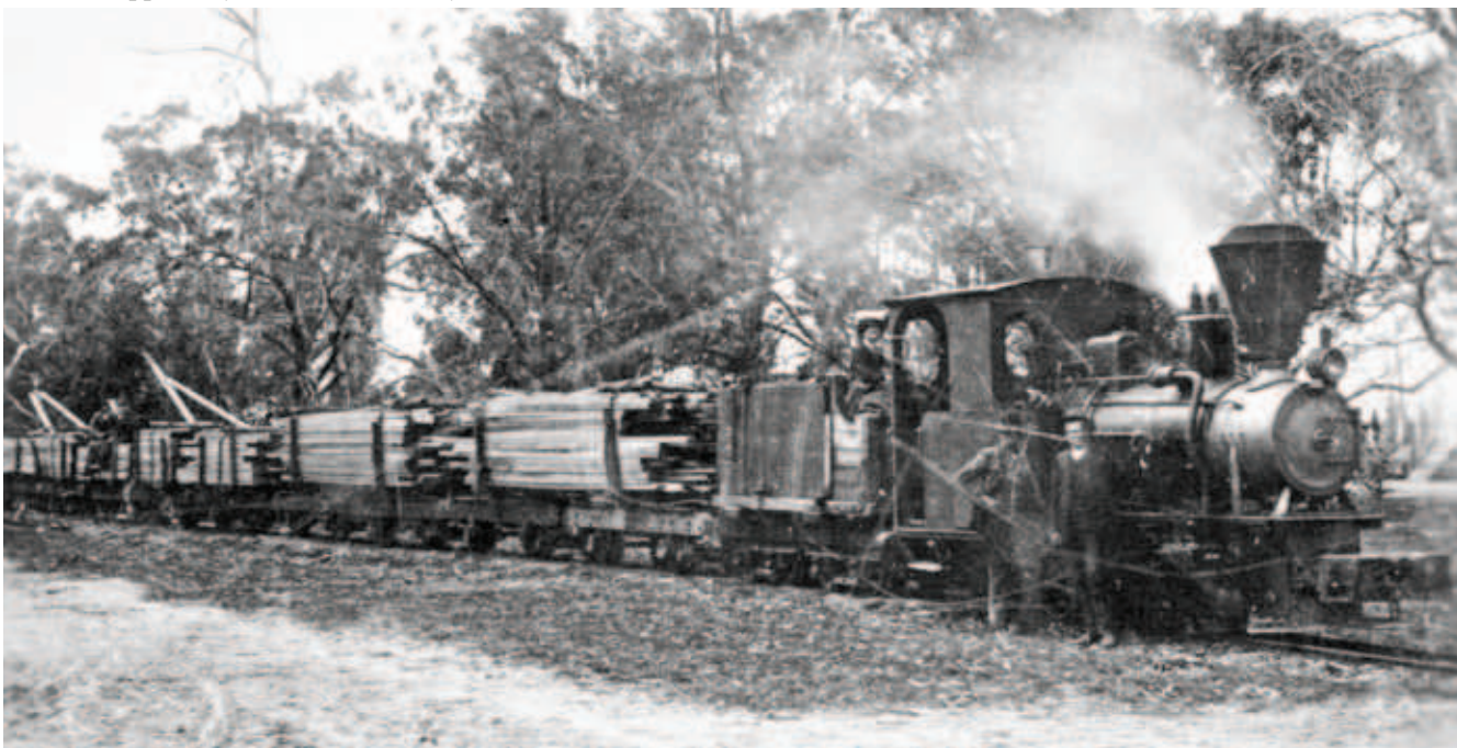
Orenstein & Koppel 0-4-0WT 'Lily' (B/No. 3771 of 1909) on the 2ft gauge Goodwood tramway at Port Albert – probably the only 2ft gauge line in Victoria built to carry logs in addition to sawn timber.
