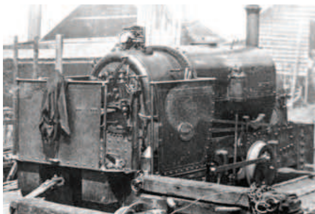
Henry's 3ft 6in gauge tramway at Forrest had tight clearances, due to a tunnel. To operate it Henry purchased a specially built loco, seen here at Henry's No.1 Mill. It was a Hunslet 0-4-0ST (B/No. 1100 of 1911) with inside cylinders and a hinged funnel.
