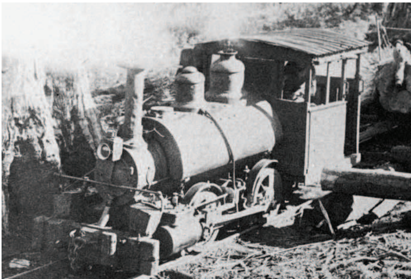
Baldwin 3ft 6in gauge 0-4-0ST (BNo. 7556 of 1885) working on the Australian Seasoned Timber Co.'s tramway at Wandong, c. 1898.
