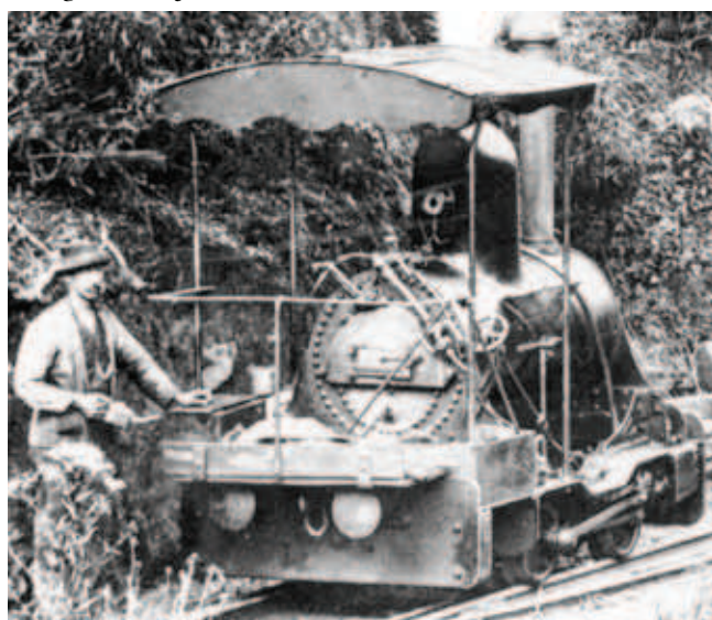
Beyer Peacock 3ft 6in gauge 0-4-0WT locomotive 'Tom Thumb' (B/No. 3057 of 1889) on Henry's tramway at Forrest. Originally built to 2ft 9in gauge it was in other respects identical to an 18 inch gauge loco Beyer Peacock built for use within their own factory. The driver is Alex McLaws. Photo: W Henry LRRSA collection
