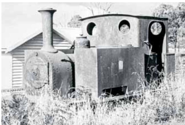
Kerr Stuart 3ft gauge 0-4-2T (B/No. 797 of 1902) abandoned at Gembrook. Photo: Andrew Lyell
