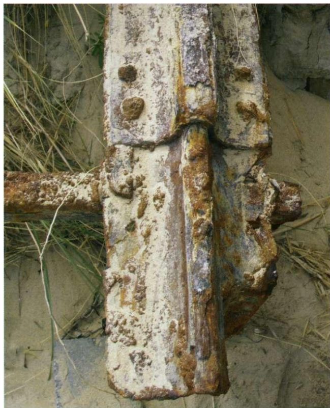
The Barlow rails at Cape Paterson were joined by connection plates. These were 32 inches in length and can be seen protruding from the end of the rail in this photograph. Photo: Mike McCarthy
